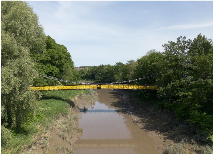
Sparke Evans Bridge and accessible ramp
