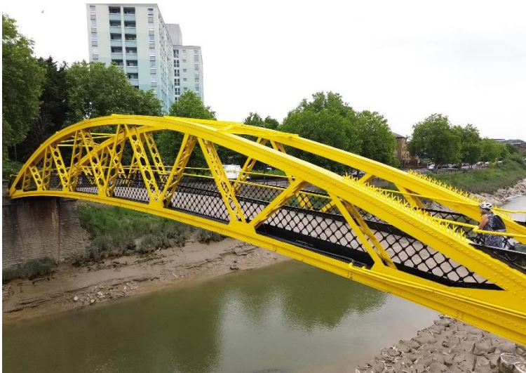
Banana Bridge (Langton Street Bridge)
