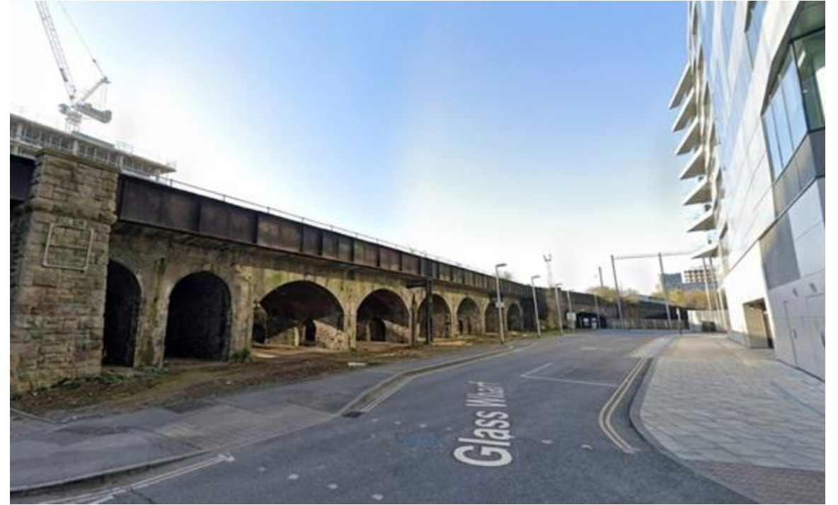
Security railings removed
