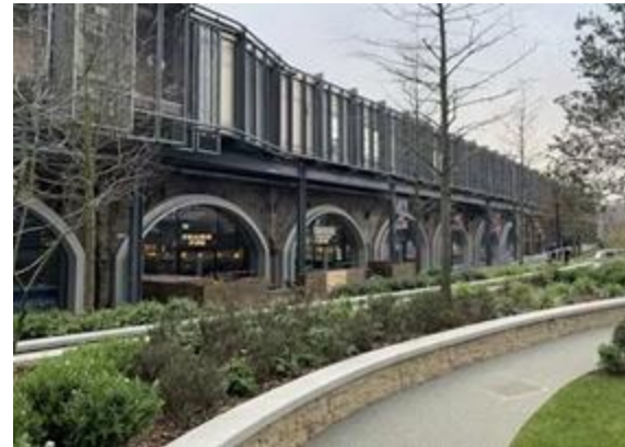
Wood Lane Arches, London
